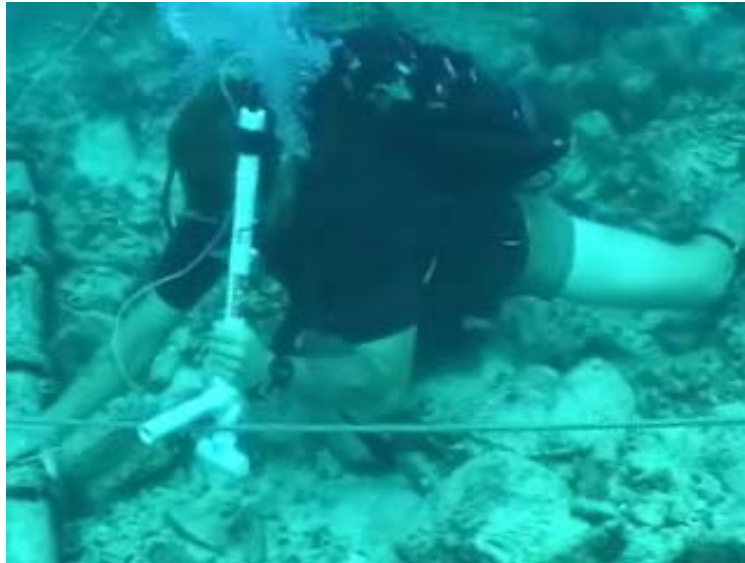
Figure 6: Tracking the Bore under the Seafloor
