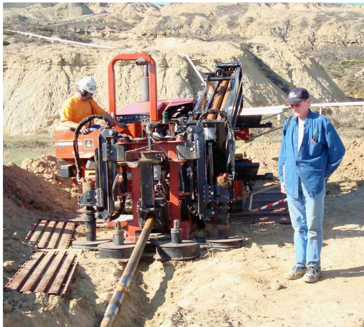
Figure 7: Ditch Witch® JT4020AT Drill Unit at Work
